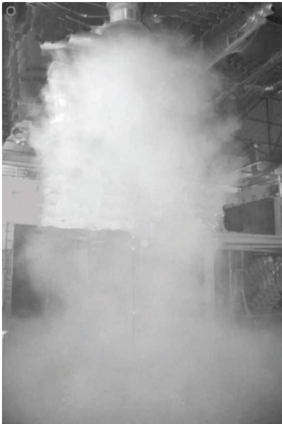
Figure 3: Smoke test in cooling
